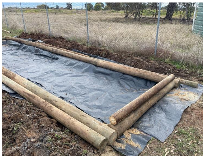
Figure 1: Construction of SPA wicking bed
